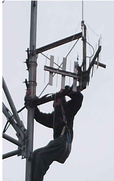
Dave—KE7YWM working on the link antenna
